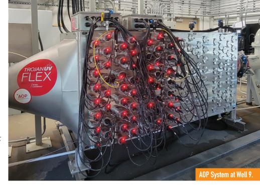
Advanced Oxidation Process (AOP) is the most technologically advanced treatment process and a proven solution that removes the compounds from drinking water. Construction of AOP reactors at Well 9 began in fall 2019, and at Well 6 in February 2020. Completion has made the wells compliant with New York State's 1,4-dioxane regulations of a maximum contaminant level (MCL) of 1 part per billion; and for PFOA and PFOS at 10 parts per trillion.
