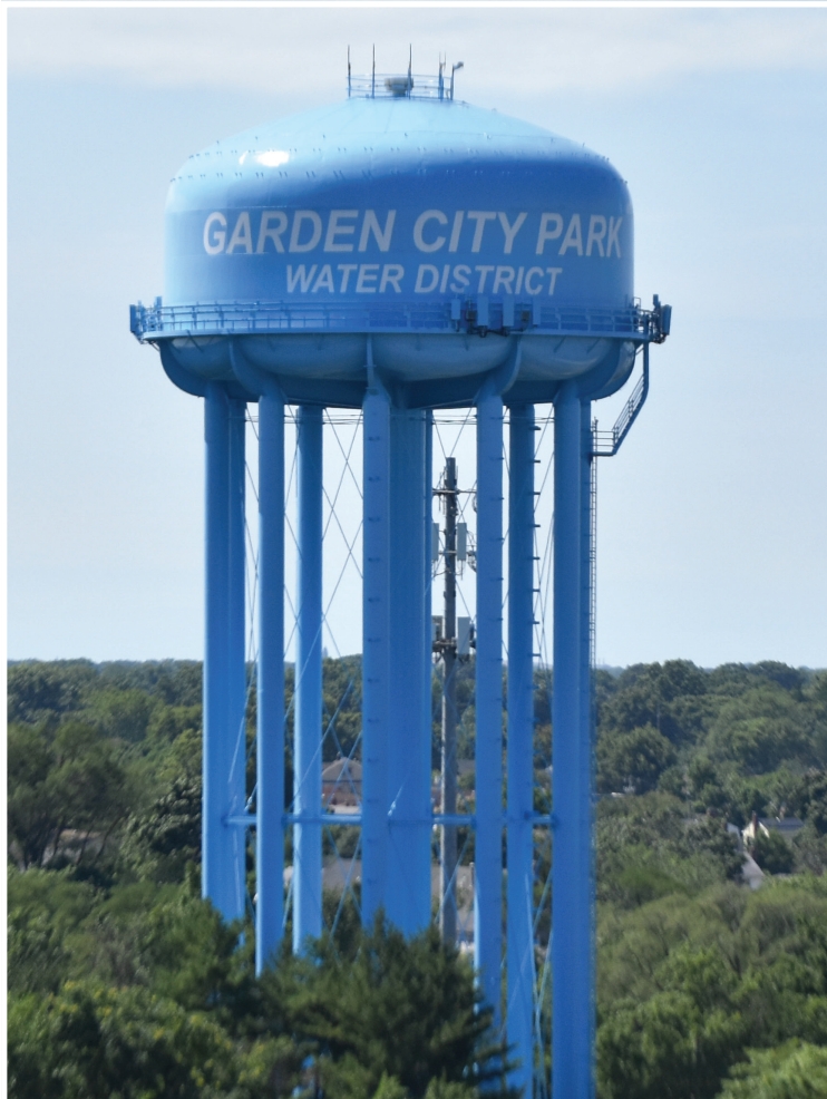
The Garden City Park trademark water tower has been freshly repainted.
